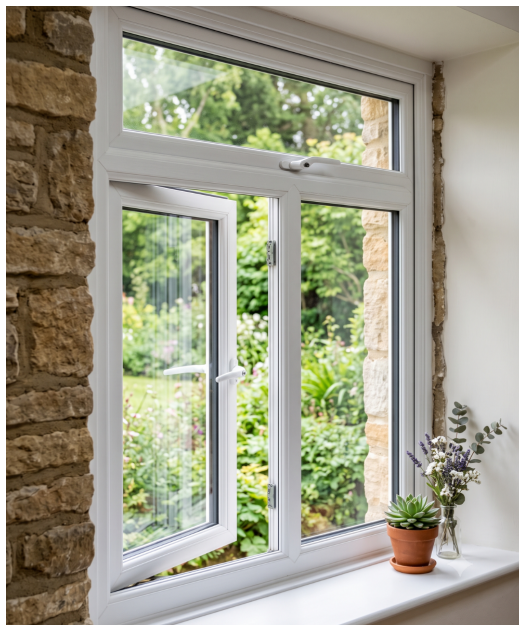
Casement UPVC windows finished in white, set into a stone facade.
