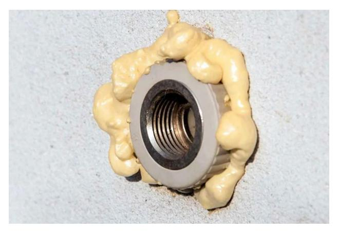
The most effective way to fill these small openings is by using off-the-shelf gap filler, while larger gaps are best blocked up with expanding polyurethane spray foam.
