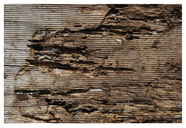
To deal with existing termite damage, remove and repair or replace any termitedamaged timber and ensure that the pests are no longer active or able to access the building. Identify the access point for any previous damage and repair or install barriers.
