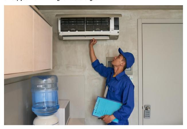
Filters are like the lungs of your air conditioning system. When they're clogged up, your AC has to work harder, which can boost energy use by 5% to 15%. A clean filter is crucial. It keeps airflow strong and improves indoor air quality. Swapping out or cleaning filters every three months, especially during peak summer months, can help your AC work better, cool faster and even keep your air fresher.
